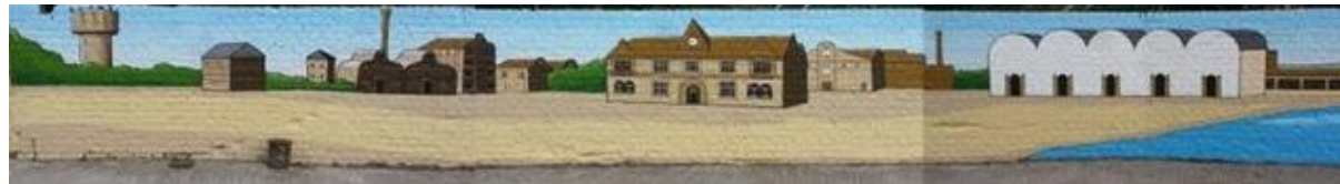
The old buildings at Sittingbourne Paper Mill
