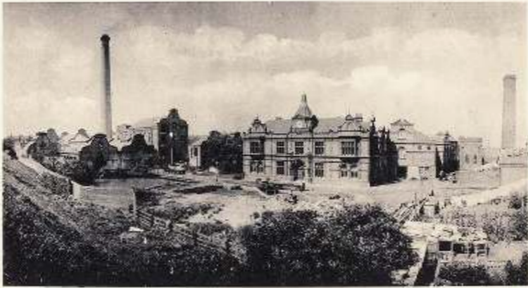
Panoramic view of the mill
